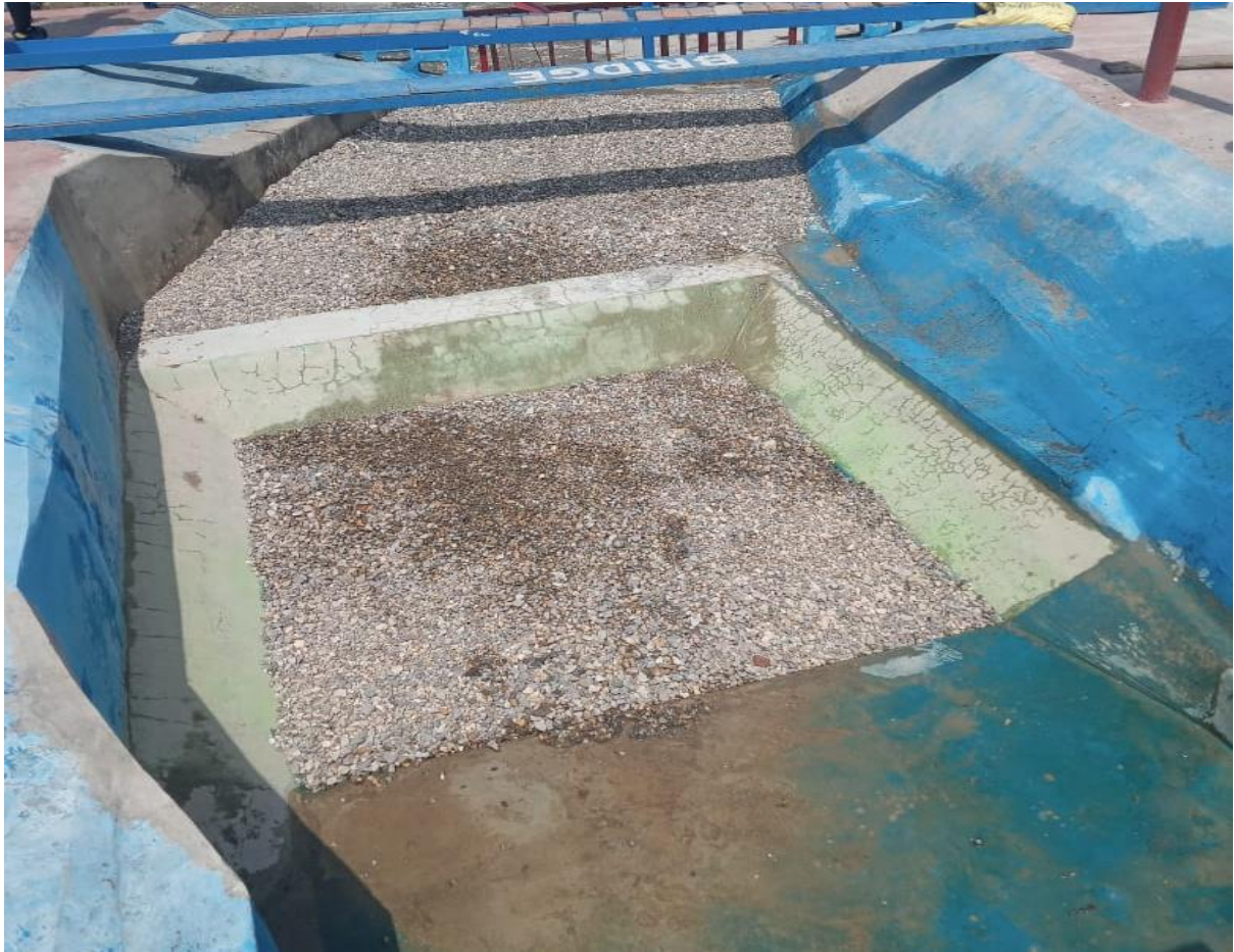
Photo 04: Dressing of Plunge pool area and downstream of Plunge pool
